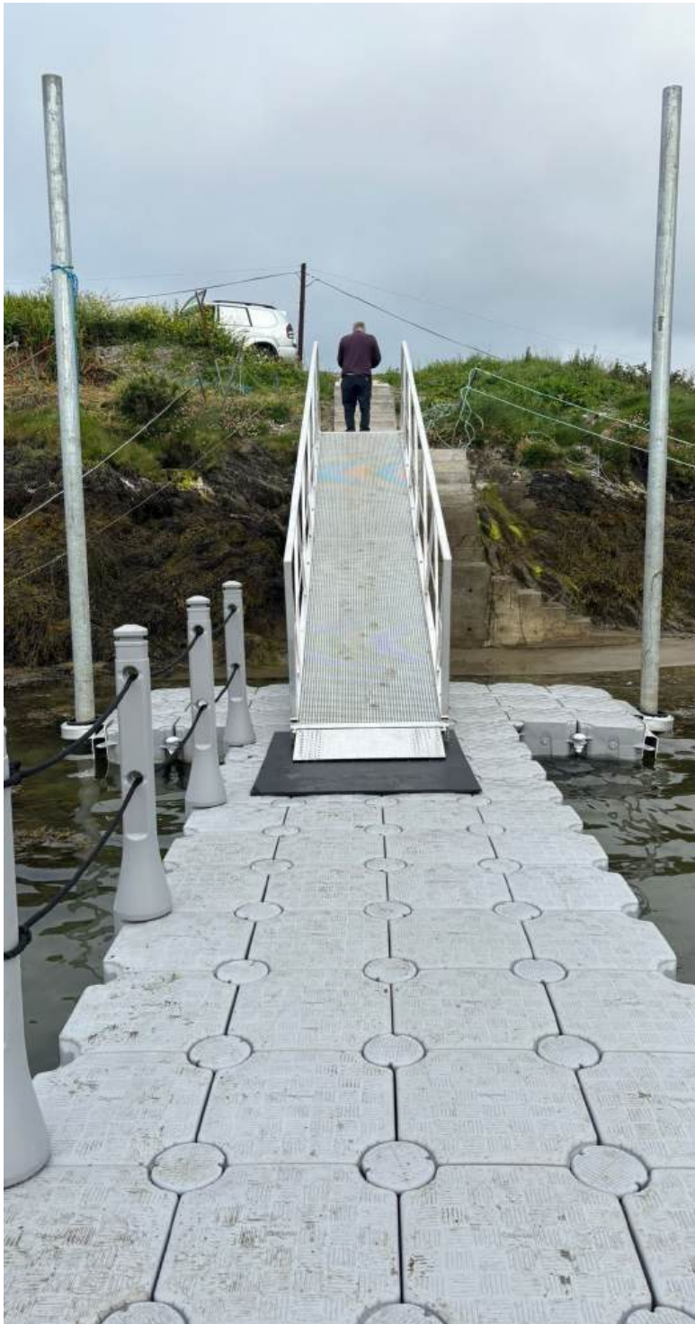
Above: The pilon system in place for this dock.
